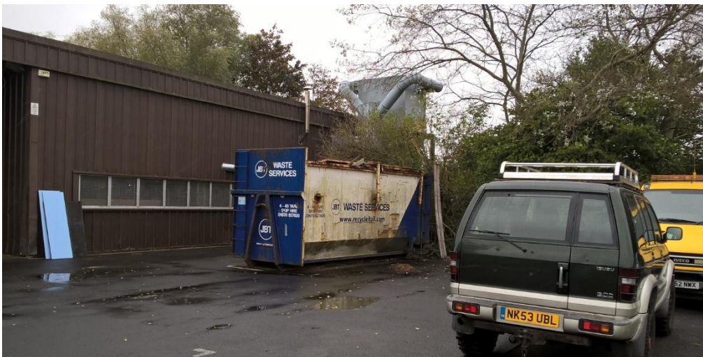
Photograph 7: Laminform Extract Plant
