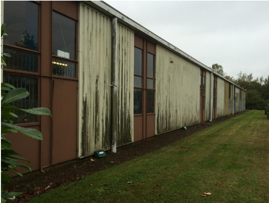
Photograph 6: Rear of MOT Premises
